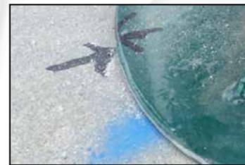
1. Place unit on concrete pad and mark holes. Mark all holes. Make a mark on the unit and the ground to make sure unit lines up with holes.
