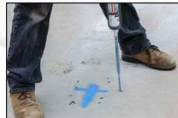
4. Fill holes with epoxy, making sure not to overfill. (Epoxy is **not** included in shipment and must be provided by installer).
