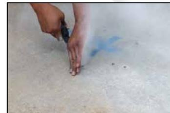
3. Using compressor or blower, blow out concrete dust from holes.
