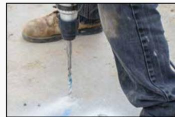
2. Drill all holes with concrete drill. Drill to a depth of 5-6" deep.
