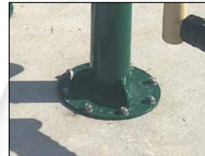
5. Place unit over holes and make sure it lines up with mark.
